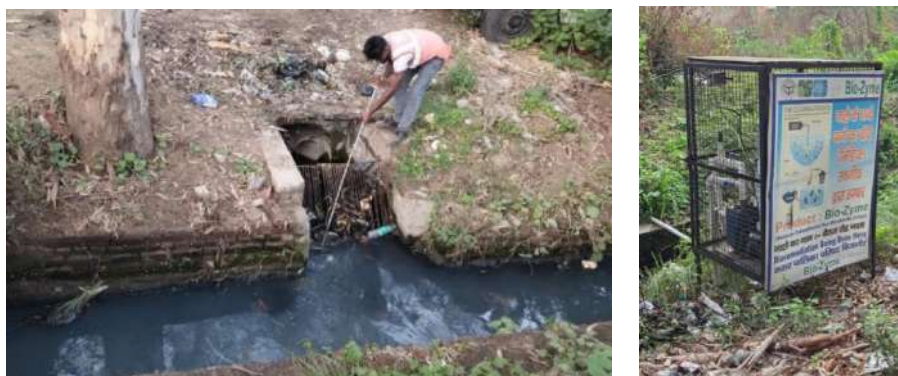
Image 4-2: Nallah Tapping and Bio-Zyme machine on Barrage Road Nallah
